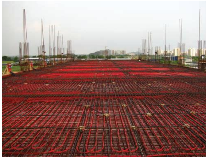
Fig. 5 Water pipes in slab cooling system [25]
