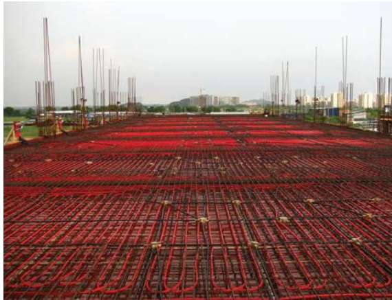
Fig. 4-5 Water pipes in slab cooling system [25][24]
