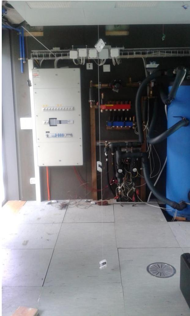
**Figure 19 Onset HOBO data loggers U12 placed at three different heights of 0.1 m, 1 m, 1.8 m for measurement of temperature and humidity**
