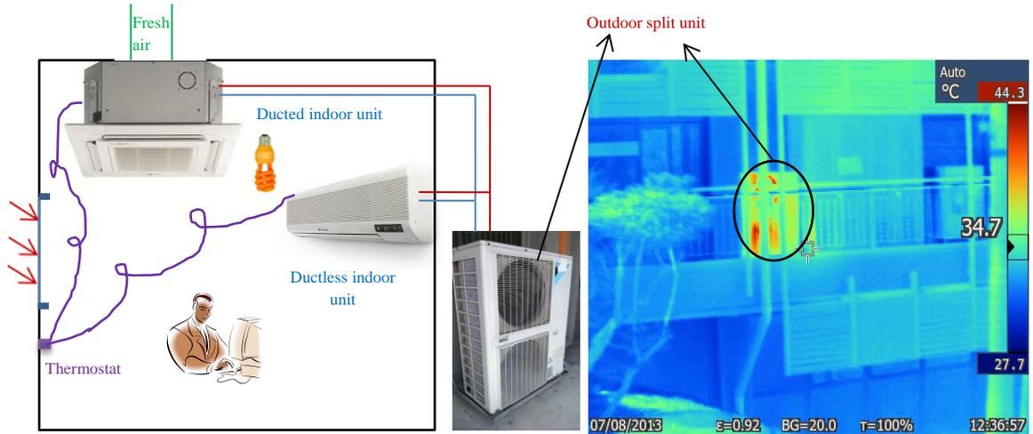
**Figure 9 Indoor and outdoor units as well as infrared image of an implemented case of split AC system**
