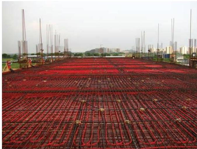
Figure 4 water pipes in slab cooling system (Sastry and Rumsey, 2014)
