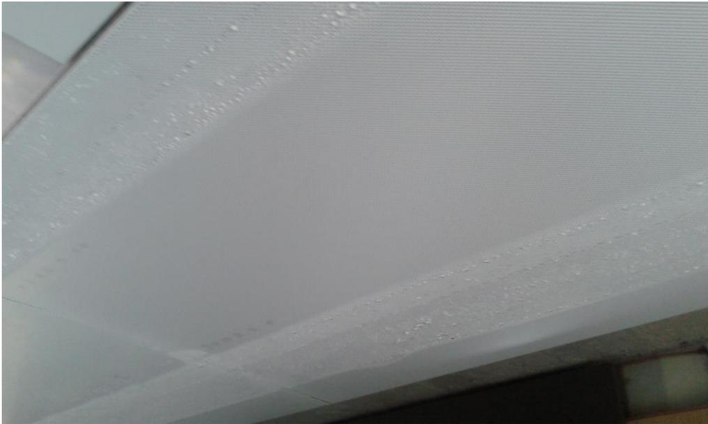
**Figure 50 Condensation pattern on the radiant cooling panel when air system is switched off**
